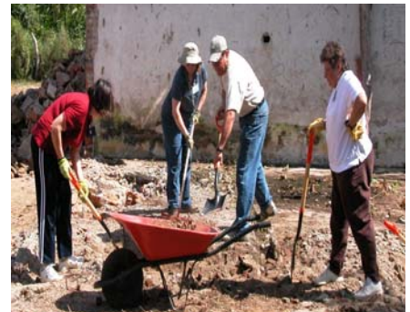
TABASCO MISSION TEAM REMOVING RUBBLE FROM FUTURE BUILDING SITE
